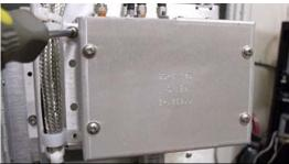
4. Reconnect the D-sub connectors to the replacement pol aux relay using a 2mm flat blade screwdriver.
