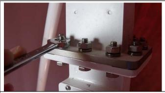
4. Install the replacement filter and LNB assembly to the feed of the system noting the alignment of the filter. No need to Loctite the threads as split washers are used on the installation.
